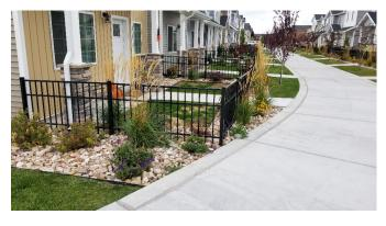
There is a metal fence enclosing each front yard. This category is not a full replacement of this fence but an allowance to refurbish the fences on a regular basis. This may include replacement of bolts, caps, and painting as needed. Full replacement of the fence has not been included in this reserve study.
