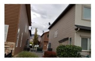
The exterior of the buildings for phase 1-3 are a combination of vinyl siding, stucco, and rock. The vinyl siding can last a very long time if it is properly maintained. Regular inspections of this component are recomended.
