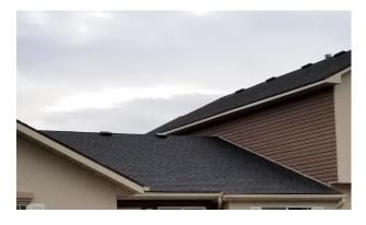
All roofs have a standard 30 year asphalt architectural shingle. Although the life of the shingle is estimated to be 30 years many factors including weather, temperature swings, ice buildup, proper ventilation can contribute to the early deterioration of asphalt shingles. This category includes phase 1-3, most of these roofs were installed between 2008 and 2012. Phase 4 has been entered as another component because most of these buildings were completed between 2015 and 2018
