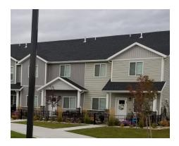
The exterior of the buildings for phase 4 is primarily vinyl siding. The vinyl siding can last a very long time if it is properly maintained. Regular inspections of this component are recomended.
