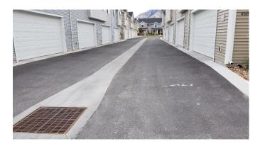
Asphalt replacement is expected to be an overlay of the existing asphalt. Regular sealing of the asphalt will help this component reach it expected life. Other factors that can cause the asphalt to fail early are, poor drainage, regular use by large trucks including garbage trucks. This category does not included replacement of concrete waterways.
