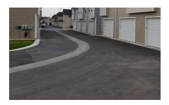
Regular sealing of the asphalt will help the asphalt reach it expected life. This estimate if for a seal coat with a 5 year life, the estimate also includes sealing of cracks with a rubberized crack filler and paiting of lines as needed.
