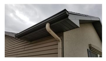
For the rain gutters and downspouts to work properly they must be maintained regularly. Regular maintenance to insure this component is clean and properly sloped is important to its proper function and overall life. When properly maintained this component may exceed it's expected life.
