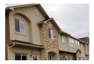
The exterior of the buildings for phase 1-3 are a combination of vinyl siding, stucco, and rock. The stucco in some areas appears to have deficiencies or that are outside the normal deterioration of this component. Be cause these issues are not spread throughout the entire community but are in specific areas this deterioration has not been factored into the estimated life of the stucco. Repairs to the stucco should be completed to help this component reach it's expected life.
