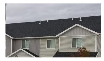
All roofs have a standard 30 year asphalt architectural shingle. Although the life of the shingle is estimated to be 30 years many factors including weather, temperature swings, ice buildup, proper ventilation can contribute to the early deterioration of asphalt shingles. This category includes phase 4, most of these roofs were installed between 2015 and 2018. Phase 1-3 has been entered as another component because most of these buildings were completed between 2008 and 2012.
