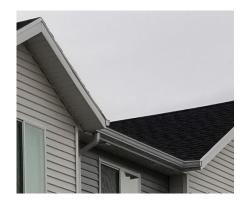
Soffit and fascia metal is composed of aluminum material with a factory white paint. Regular
